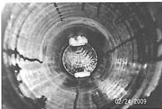
Water flowing from perimeter drain at sampling port
