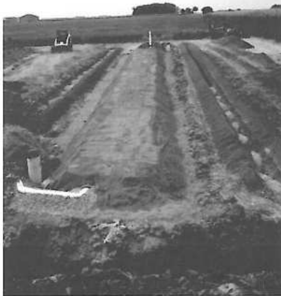
Absorption bed with perimeter drain installed
