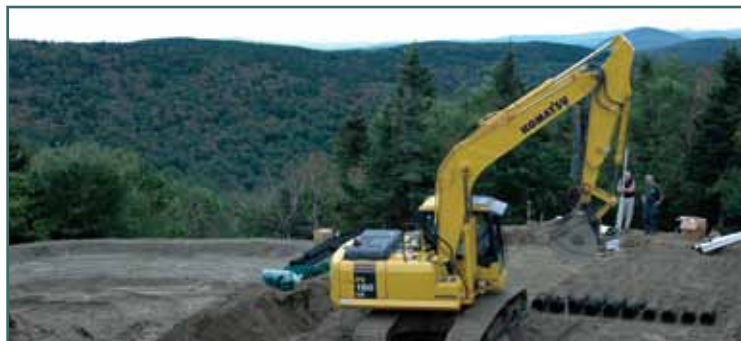
Halfway through the placement of the pipe.
