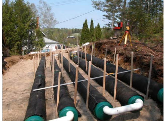
Enviro-Septic® on sloping terrain
