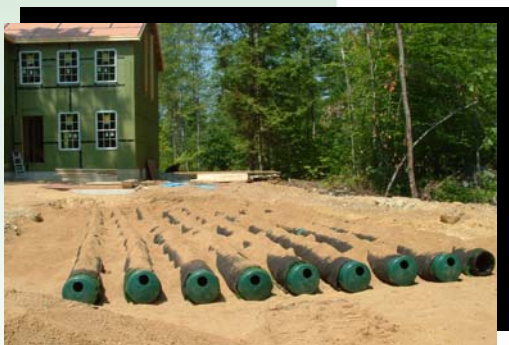
Enviro-Septic® Installation at LEED Certified Home
