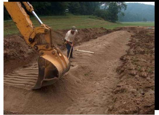
Enviro-Septic® Installation in Indiana
